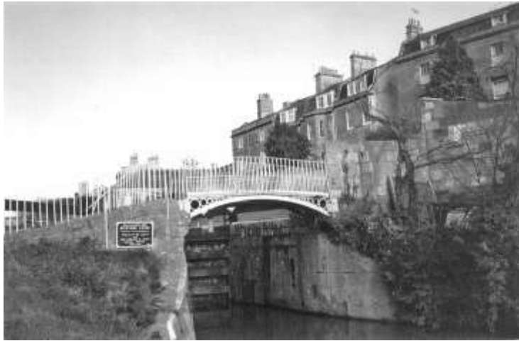
Above. Stothert Bridge over the Kennet & Avon Canal
