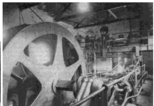
The engine before it was dismantled
